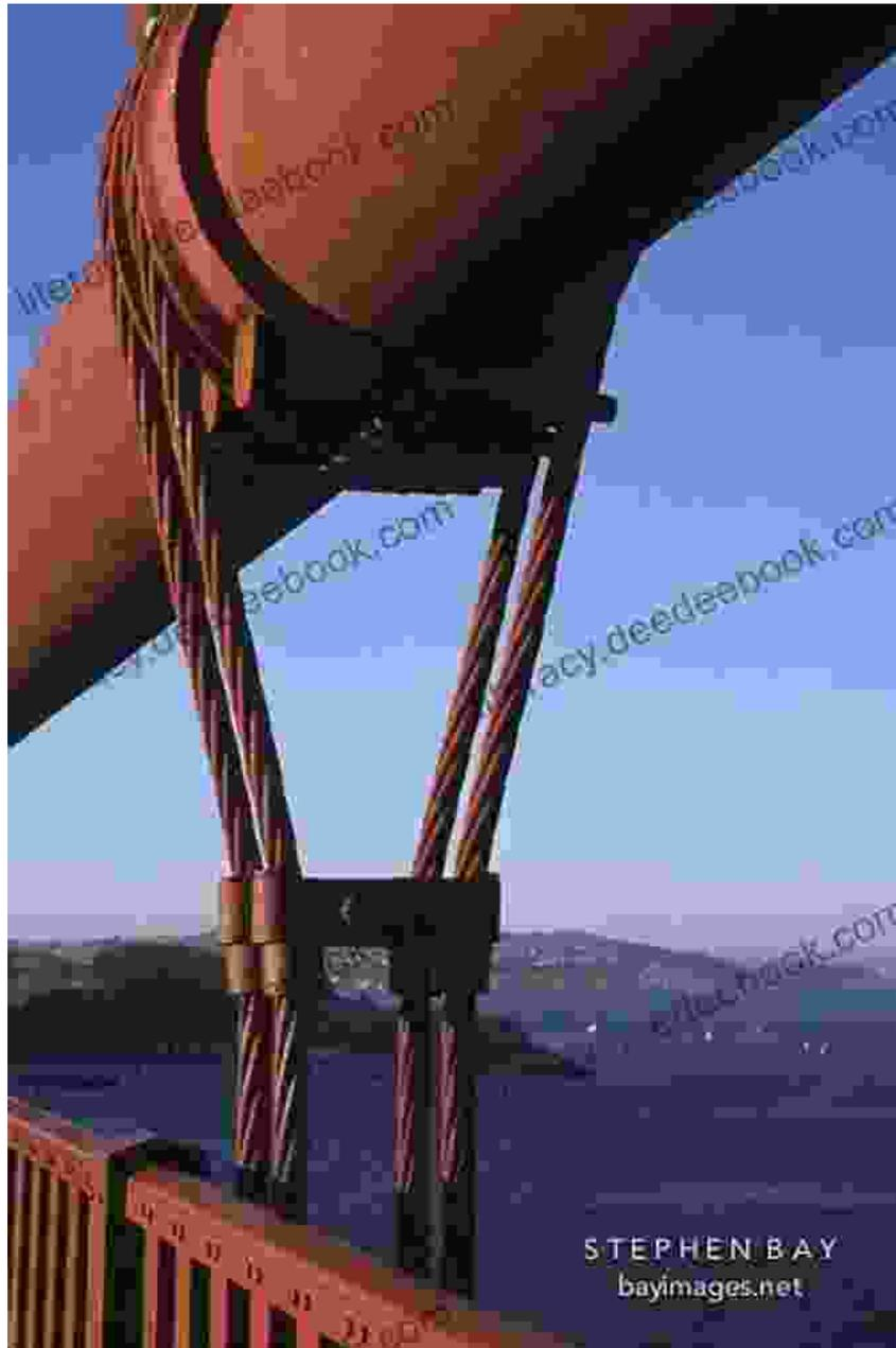
The Golden Gate Bridge is a marvel of engineering. Its suspension towers soar to a height of 746 feet (227 meters), and its suspension cables, each composed of 27,572 individual wires, span a distance of 4,200 feet (1,280
